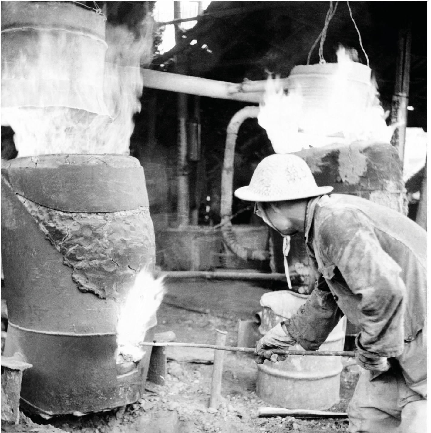
Figure 3.4: An example of the 'backyard' furnaces constructed during the Great Leap Forward.
