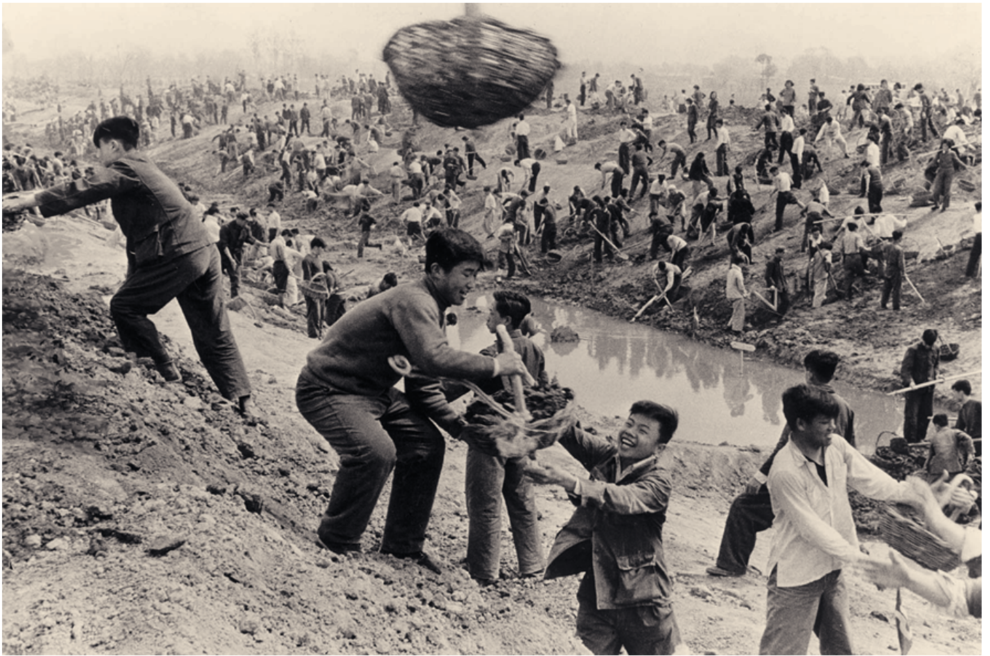
Figure 4.1: Commune members building the Sanmenshia Dam during the Great Leap Forward, 1958.
